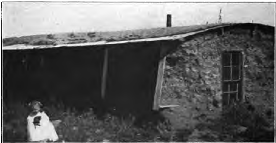
A SOD SHANTY In Buildings Such as These Many of Jackson County's Pioneers Had Their Homes.
