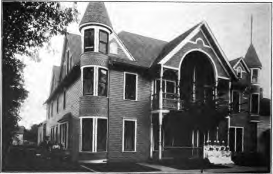
SOUTHWESTERN MINNESOTA HOSPITAL, HERON LAKE
